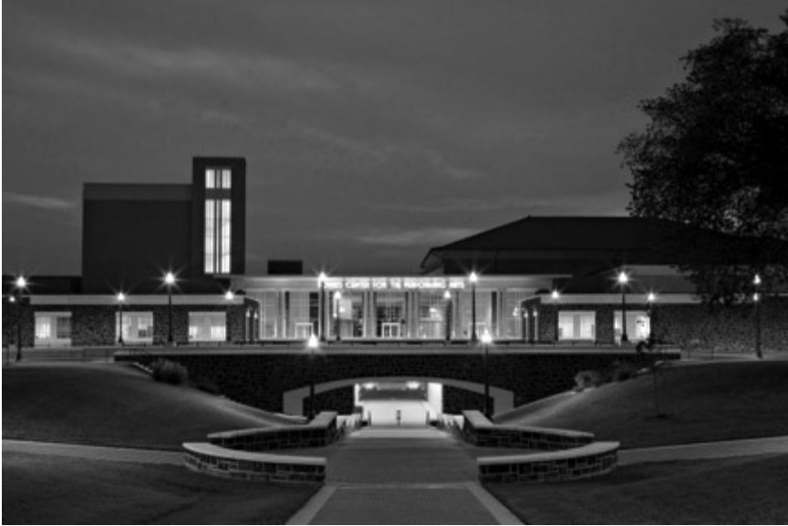
©2010 ROBERT BENSON PHOTOGRAPHY Site challenges were overcome by the tunnel connection under a major city street and U.S. highway. Nestling the Concert Hall platform, orchestra pit and student practice rooms into the sloping grade allowed for a central grand lobby.
