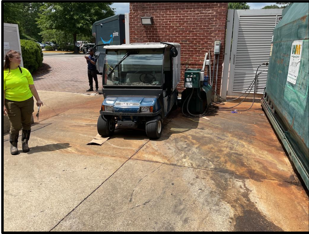
Photo #5: Rust stains and discharge from trash compactor
