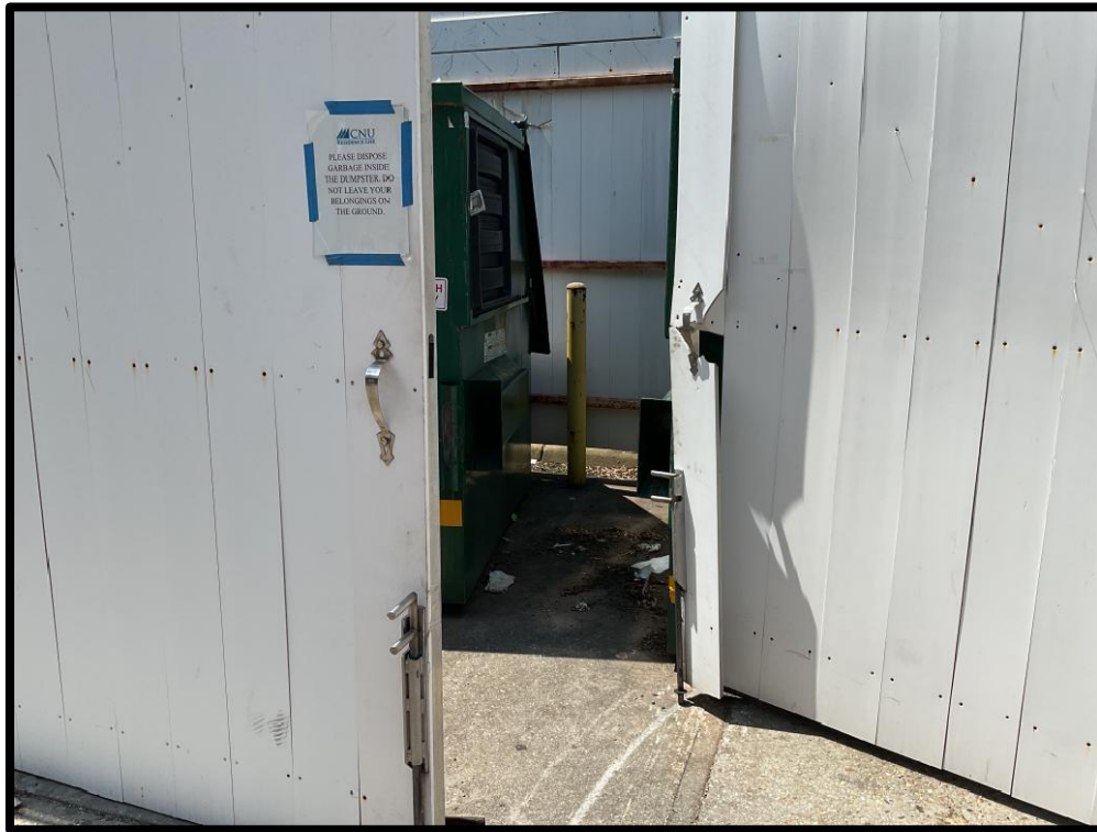
Photo #3: Some trash and debris present around receptacle area
