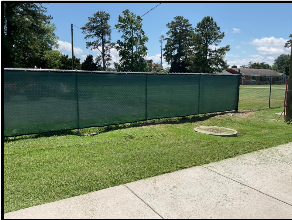
Photo #1: Grate inlet
