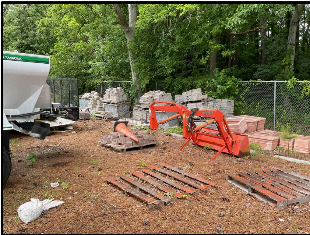
Photo #12: Uncovered materials storage
