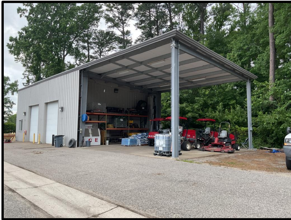
Photo #9: Covered equipment, materials, and storage area
