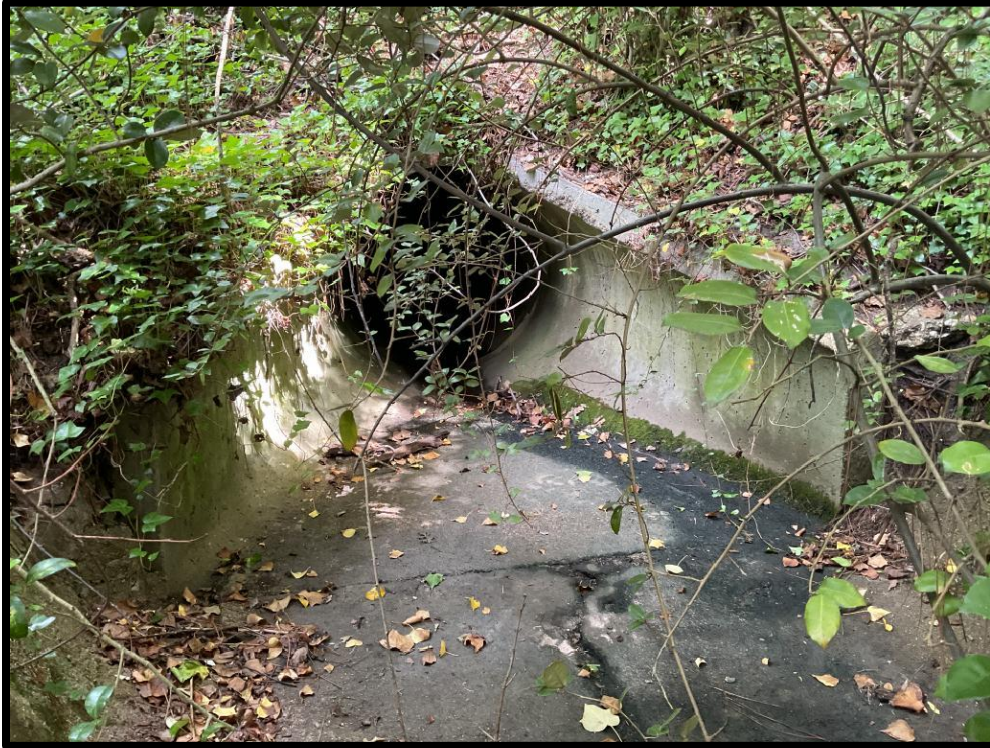
Photo #1: 24" Concrete pipe
