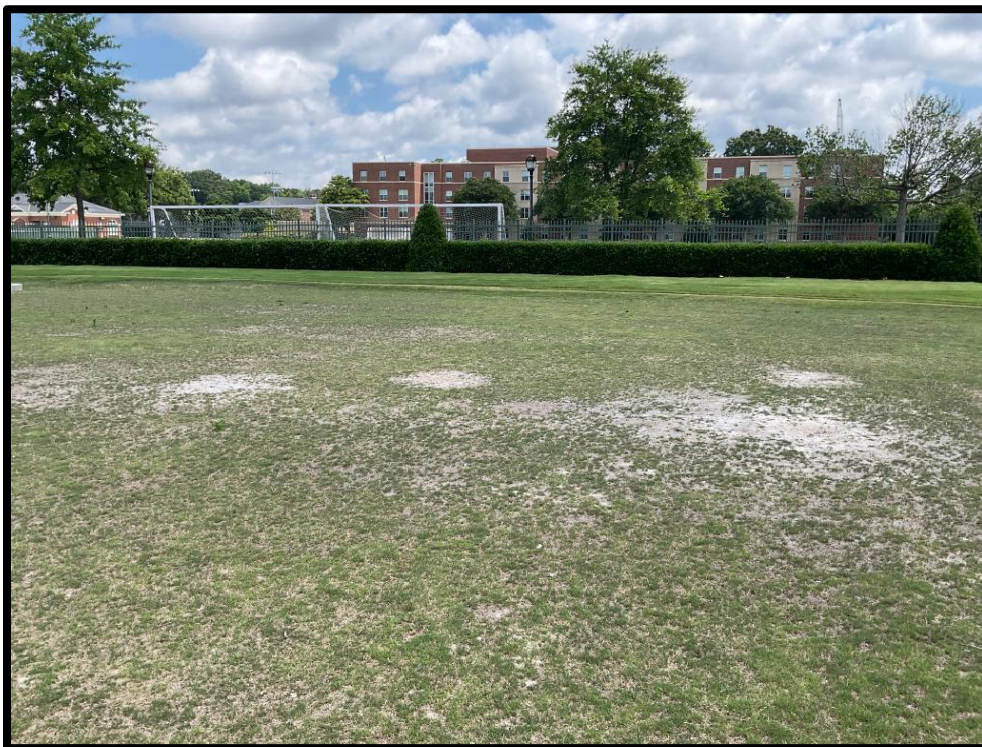
Photo #2: Bare areas present in Bioretention
