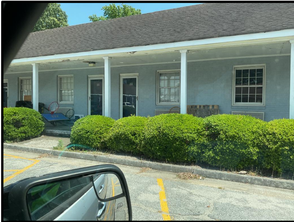
Photo #3: Covered materials storage present
