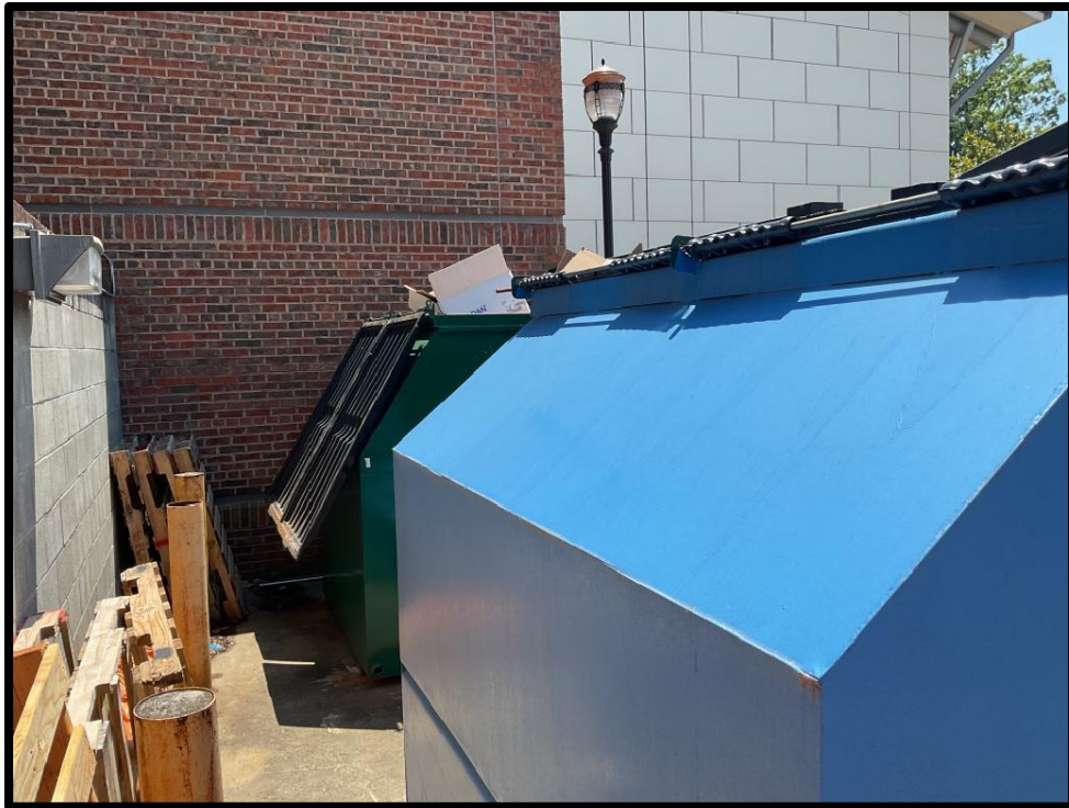
Photo #1: Uncovered dumpster
