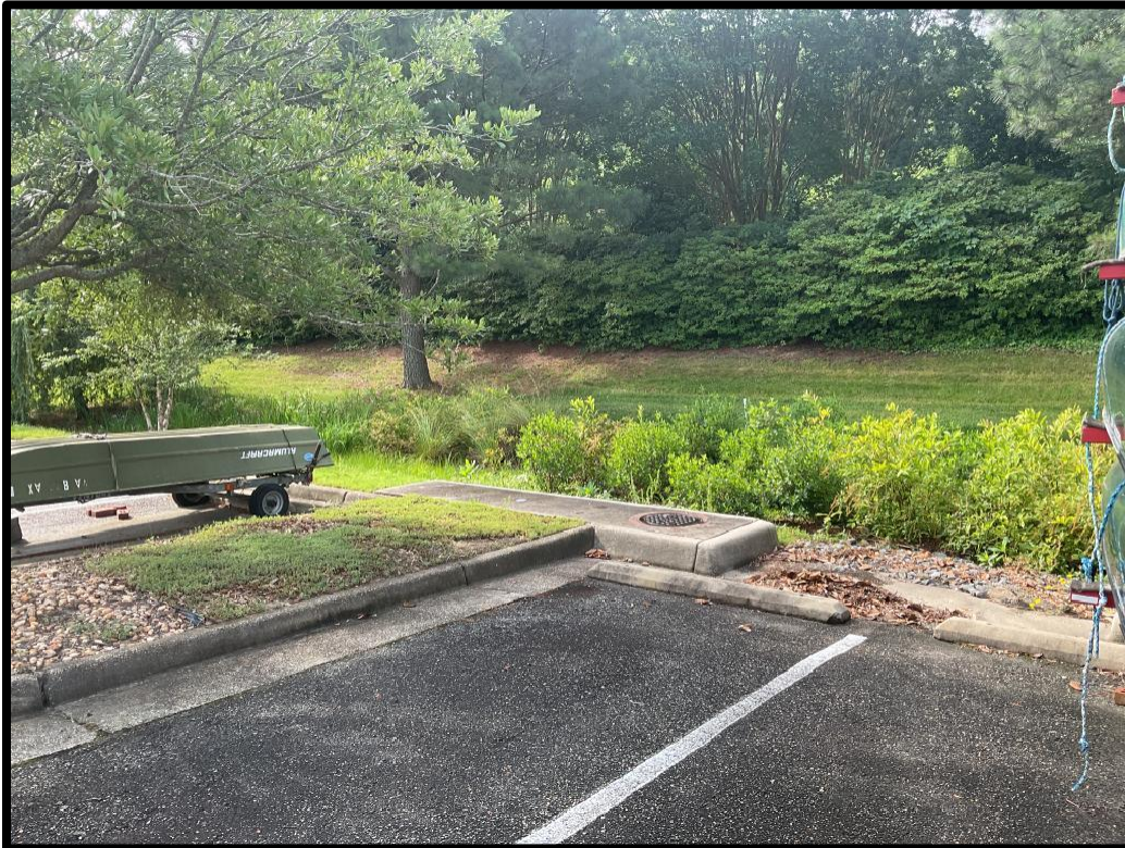
Photo #3: Some debris and road grit accumulation present in northern curb cut inlet
