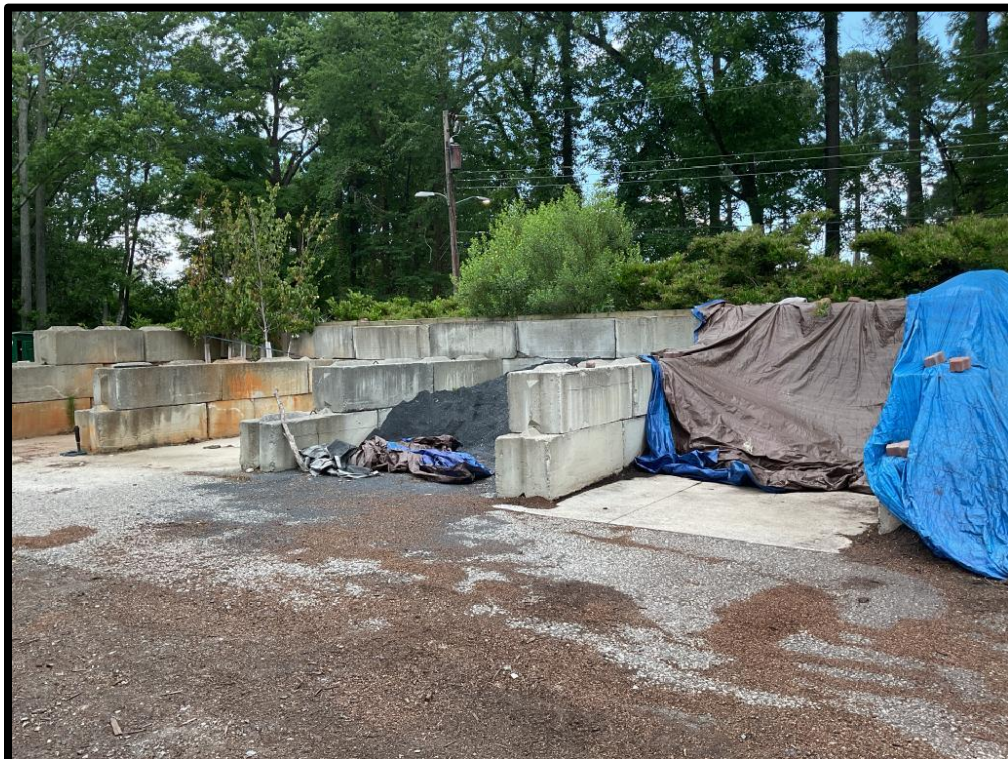
Photo #2: Partially covered and contained stockpiles
