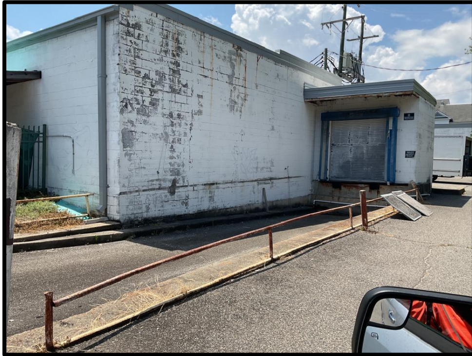
Photo #5: Loading/Unloading Area
