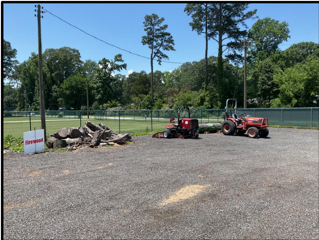
Photo #8: Work in progress near dumpster area
