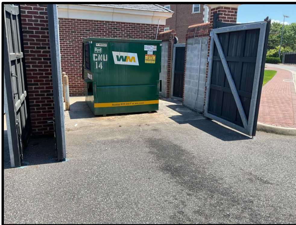
Photo #2: Uncovered dumpster
