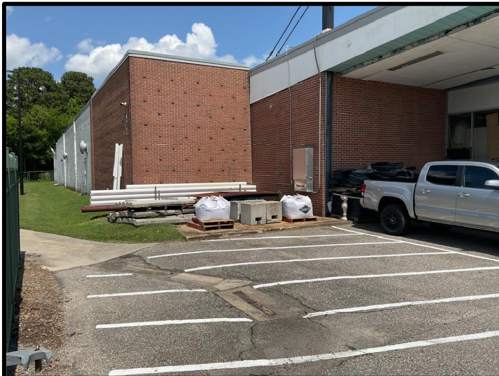
Photo #2: Uncovered material storage area
