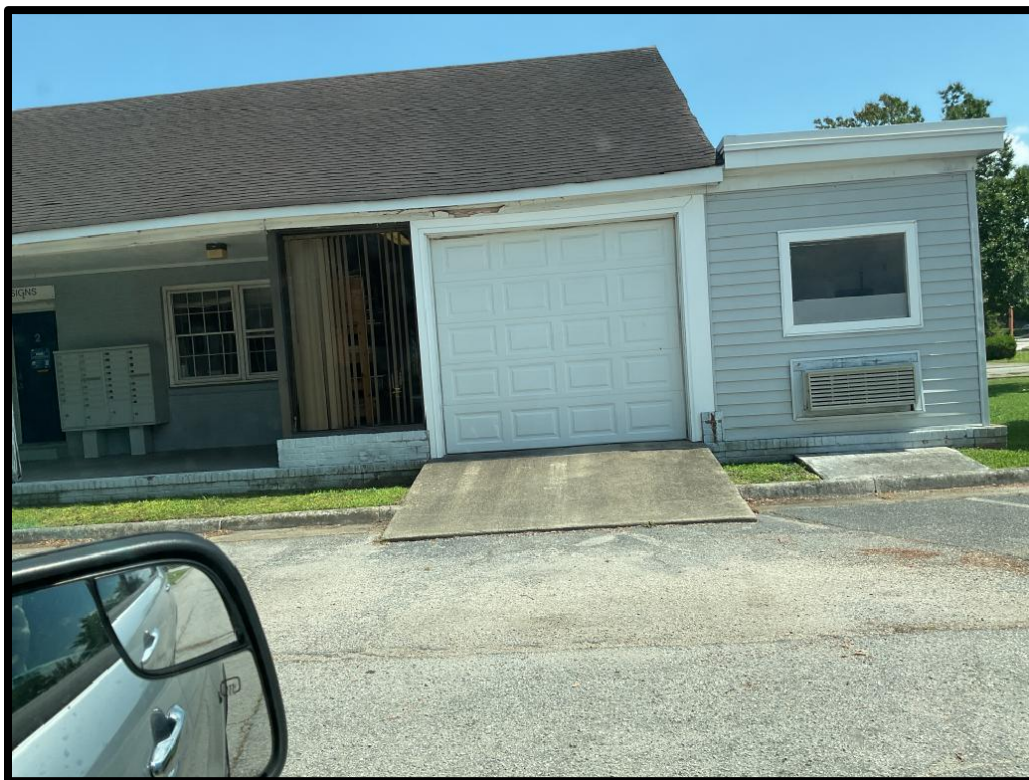
Photo #4: Loading/Unloading Area
