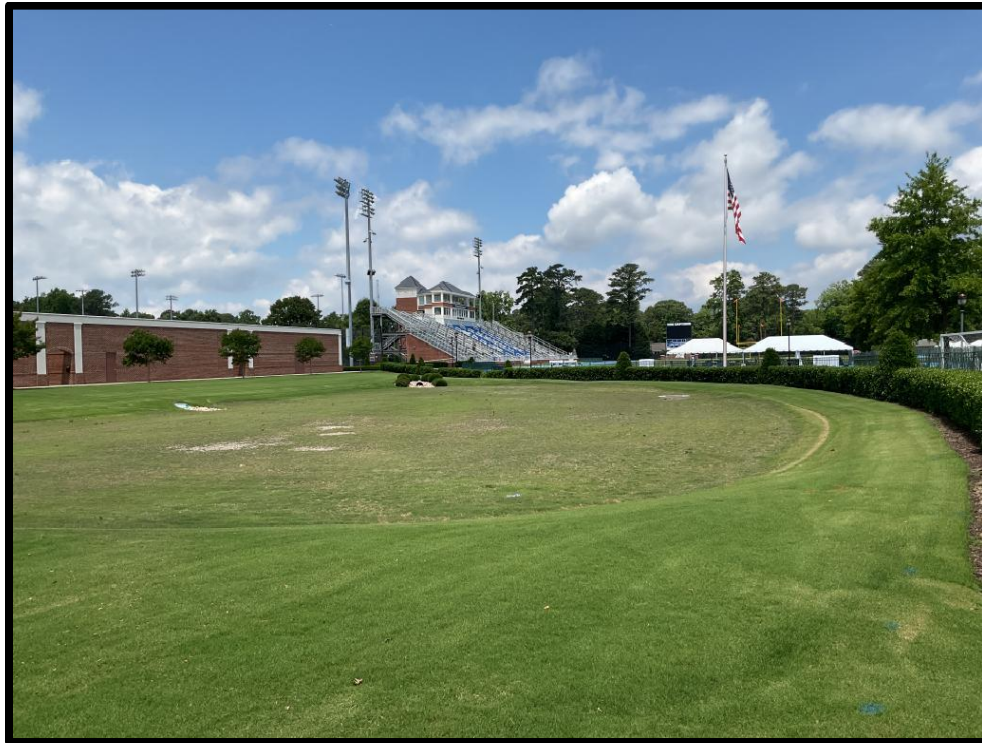
Photo #1: Overall of Bioretention
