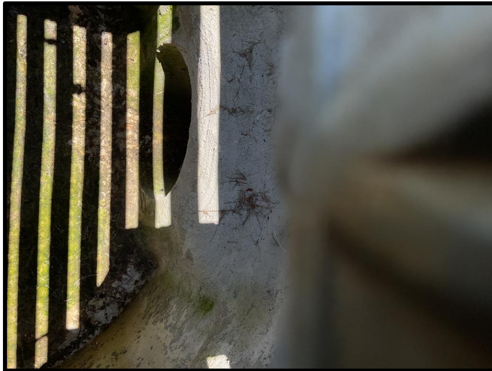
Photo #2: Upstream outfall pipe
