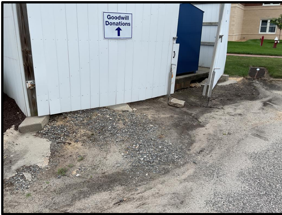
Photo #1: Significant road grit accumulation outside of receptacle area
