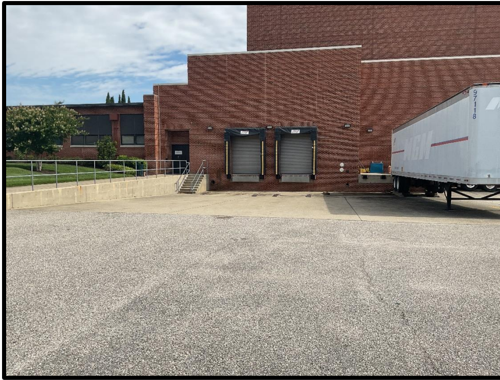
Photo #1: Loading/Unloading Area
