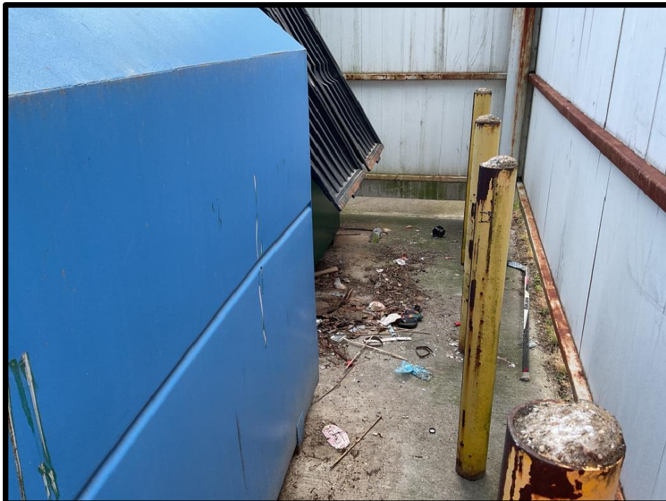
Photo #2: Trash and debris present around receptacle area
