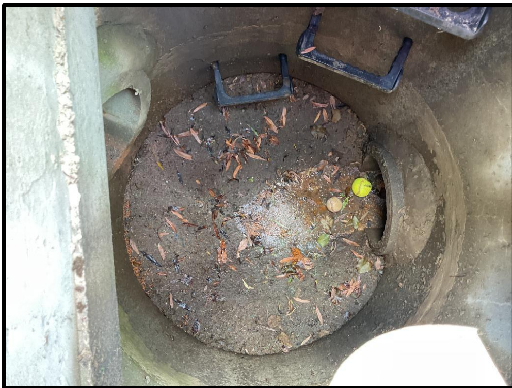
Photo #2: Some sedimentation and debris accumulation present
