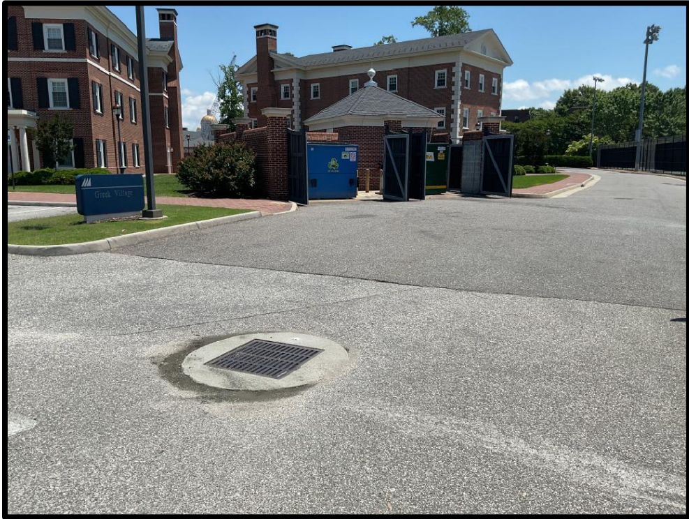
Photo #3: Stormwater inlet near receptacle area
