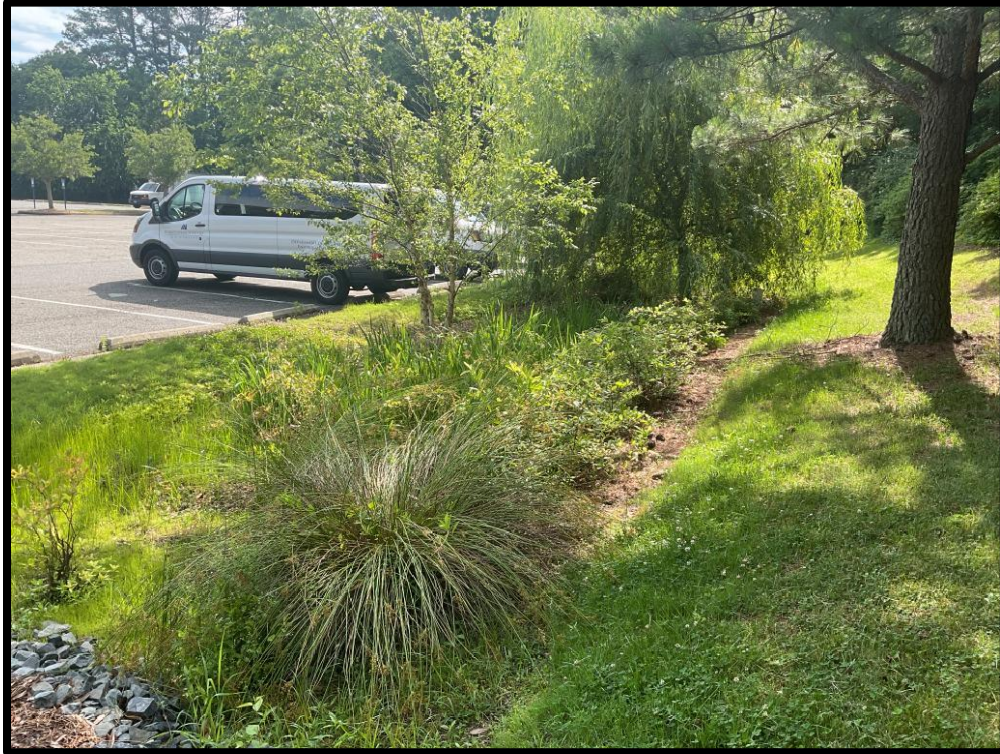
Photo #1: Overall of Bioretention
