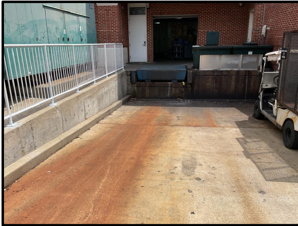
Photo #1: Loading/Unloading Area
