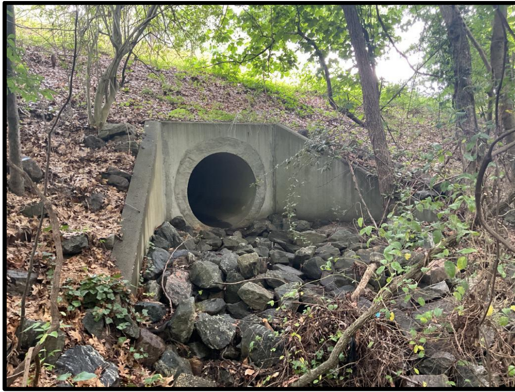
Photo #1: 48" Concrete Pipe
