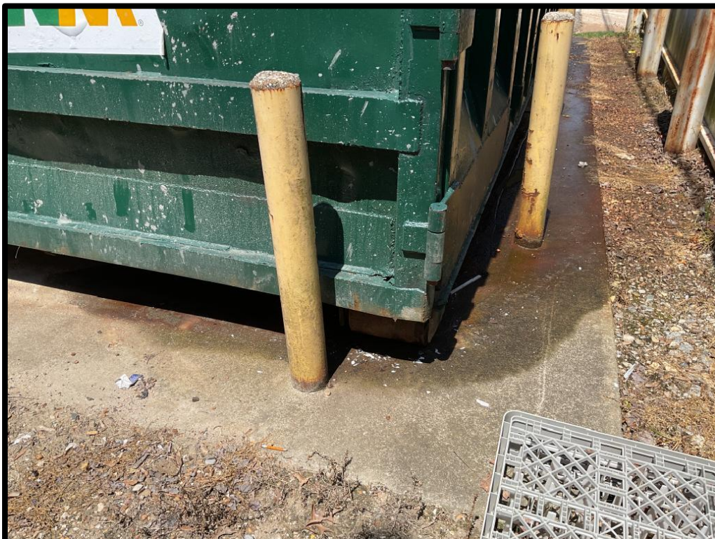
Photo #8: Rust stains and active discharge from dumpster
