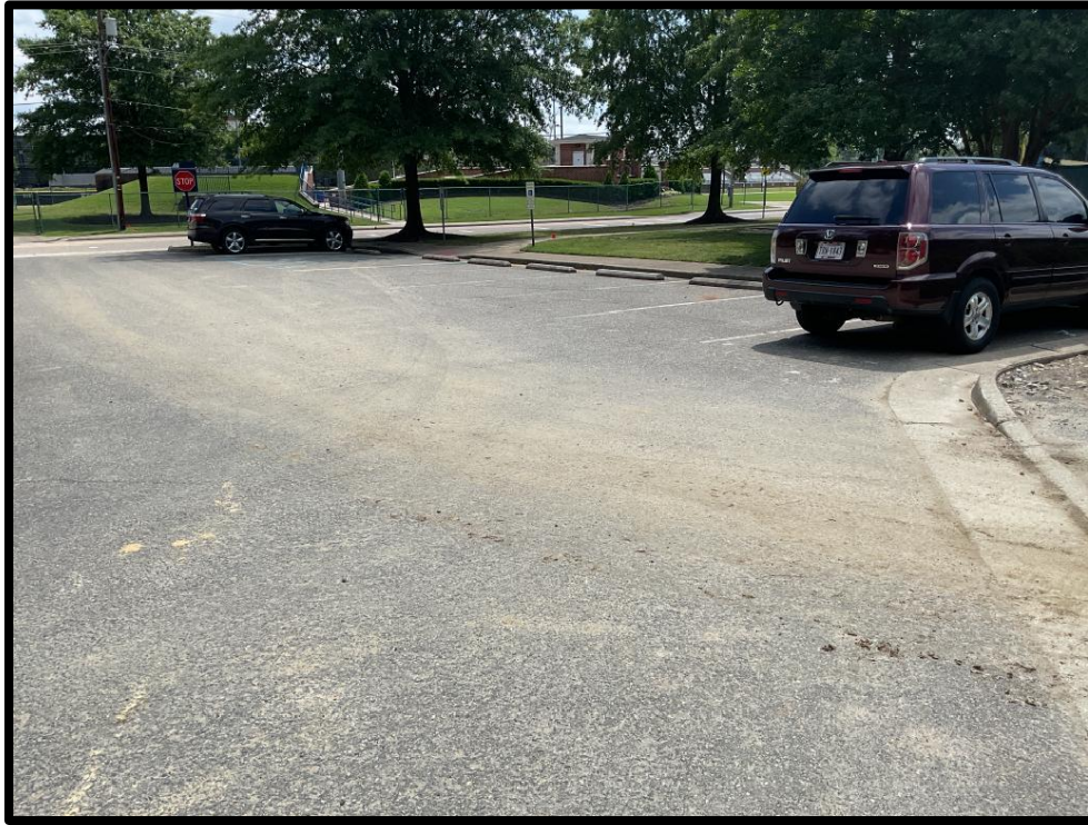
Photo #3: Sediment tracking onto parking lot from active baseball field operations
