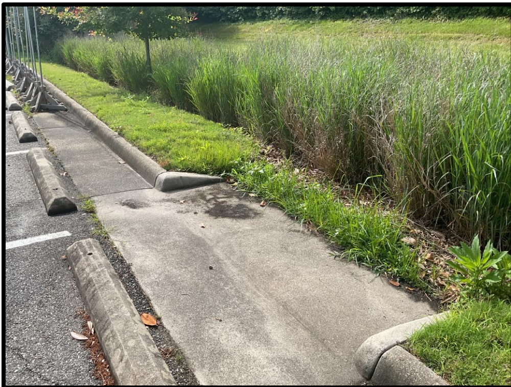
Photo #2: Some road grit and overgrown accumulation present in northwestern curb cut inlet
