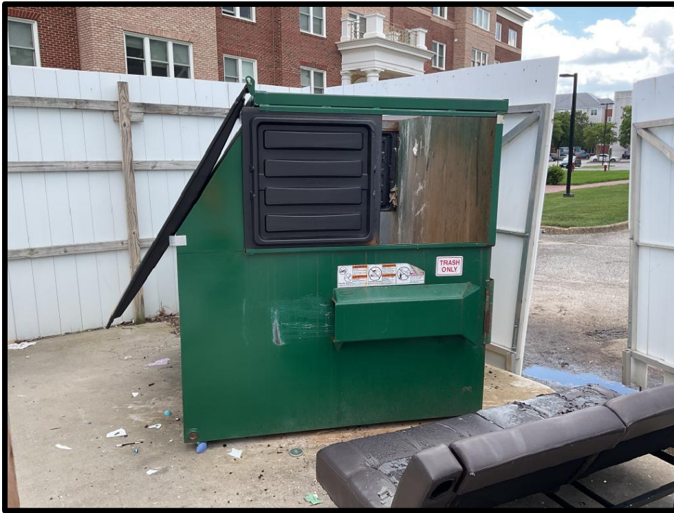
Photo #1: Uncovered dumpster
