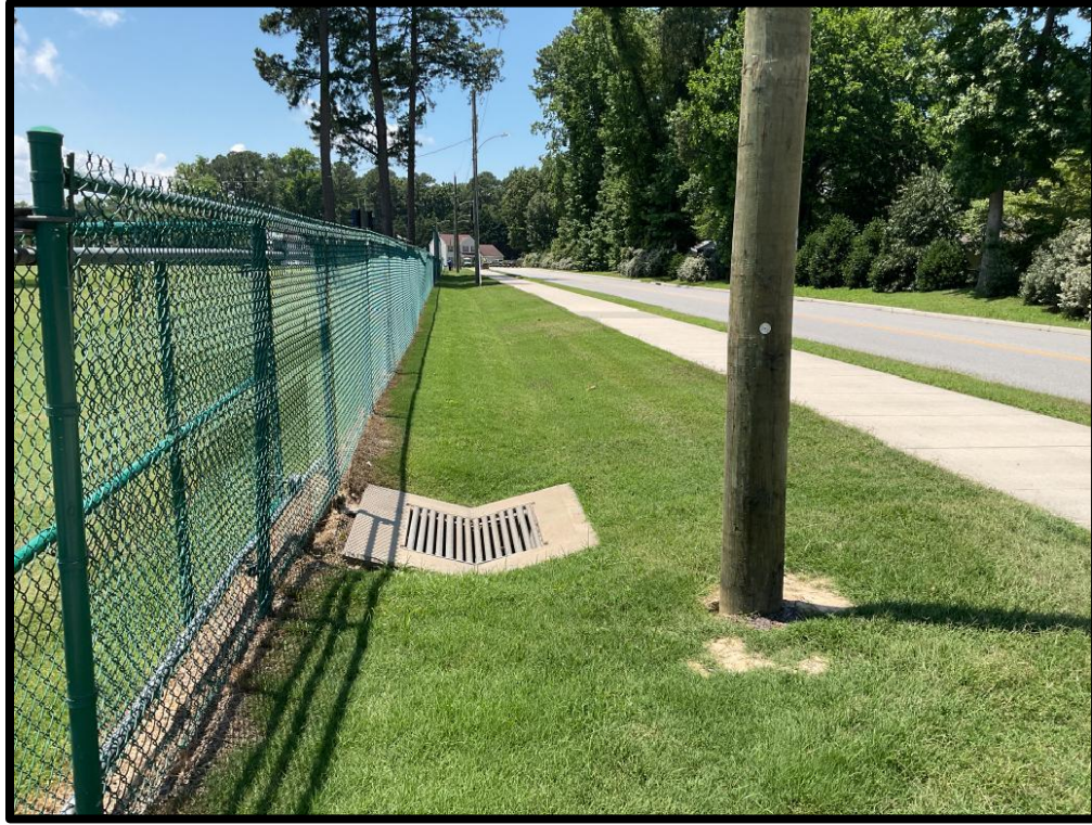
Photo #1: Grate channel and grate inlet
