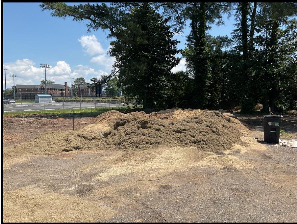
Photo #7: Work in progress near dumpster area
