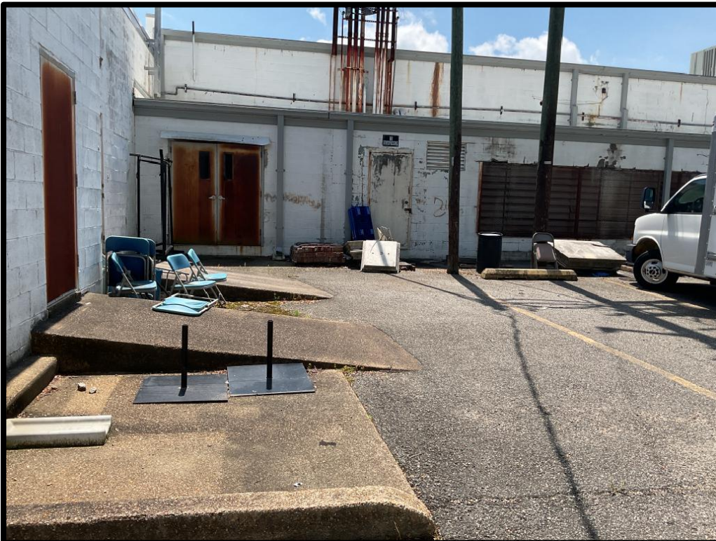
Photo #4: Uncovered materials storage area
