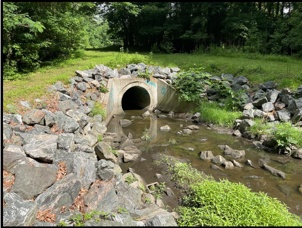
Photo #1: 72" Concrete Pipe
